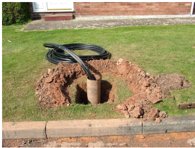
(B) Vertical Drilled Borehole
